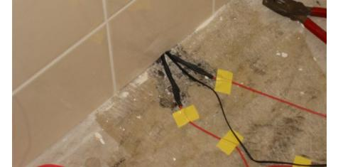
⇒ Once the cold tails are pulled up through the wall, element integrity tests to be performed
