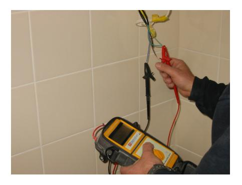
$\Rightarrow$  Attach the element tester as instructed
