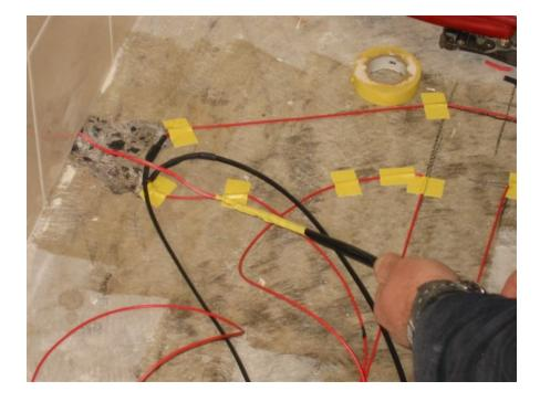
⇒ Ensure that the cold tails are recessed into the floor
